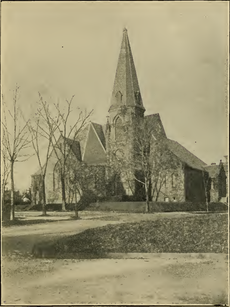
FIRST PRESBYTERIAN CHURCH, PASSAIC, NEW JERSEY.
